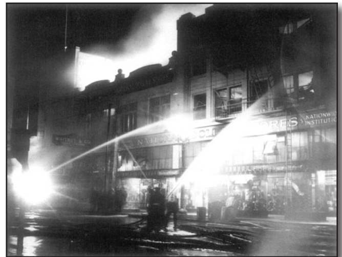
Figure 1-15 Whitney Department Store Fire
